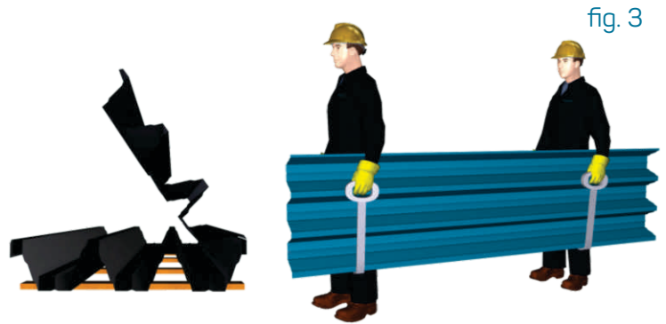
The fixing equipment, as well as the gloves must be cleaned, so that they do not damage the panel surface.
