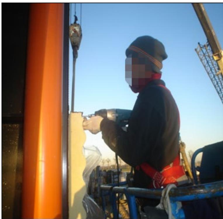
The horizontal Isoclass panel installation system entails using a crane, required to position the panel, and two basket cranes with relevant operators to assist in positioning and fastening.
