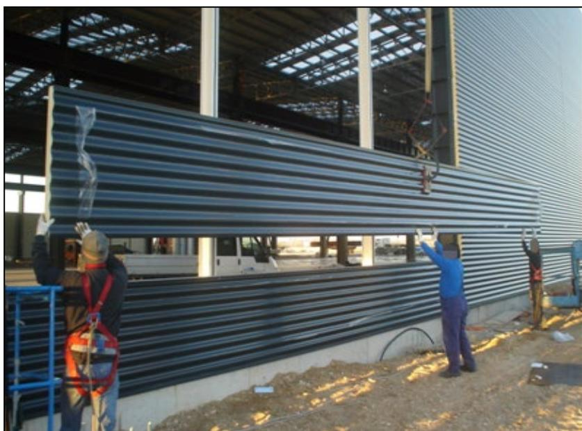
Lay the panel onto the structure and slide it down until it fits into the lower panel. Pay the utmost attention to parallelism with the structure and to ensure the wall is plumb.
