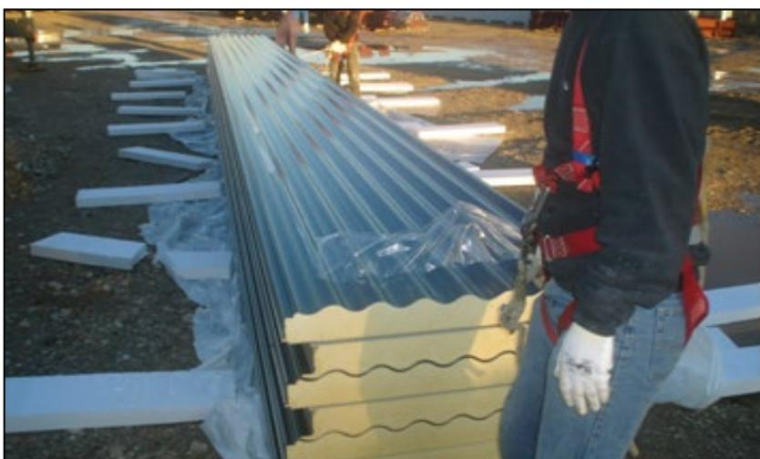
Turn the edge panel, and hook it with a clamp, prepared with the suitable moulded pad supplied by Isopan S.p.A.
